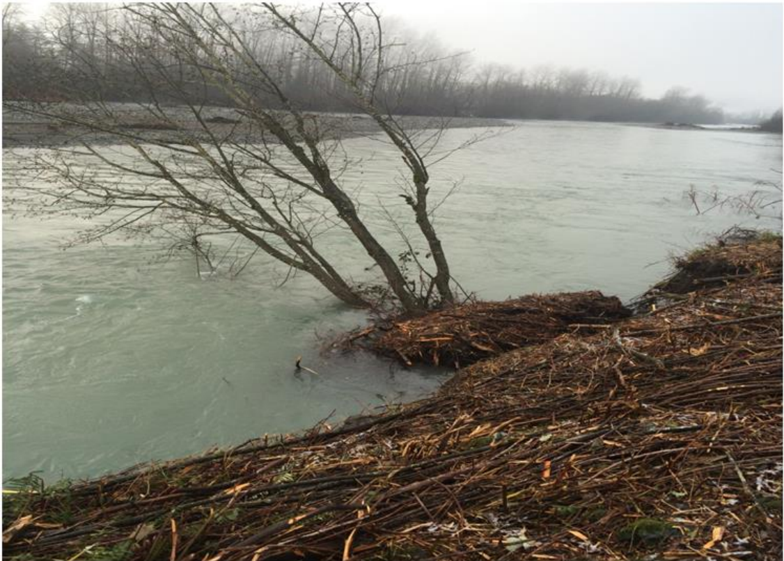
(photo of erosion area prior to repair)
