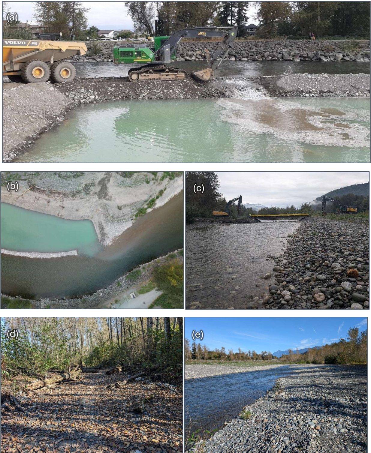
Figure 11. Photos taken at Giesbrecht Bar by environmental monitors. (a) Excavator pausing at downstream end to allow pit to fill and water levels to equalize (Sep 13, 2024). (b) Flow of turbid water from the pit following pit openings on Sep 13, 2024. (c) Bridge removal during light rain on Sep 13. (d) Restoration of pre-existing access road through the riparian area (Oct 11, 2024). (e) Site of first bridge crossing after restoration was completed (taken Oct 11, 2024).
