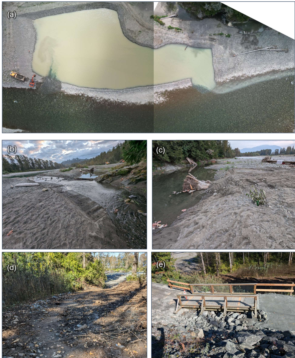
Figure 7. Photos taken by environmental monitors at S45 Bar. (a) Aerial image of S45 with turbid water slowly flushing out of the pit (Sep 12, 2024). (b) Restored trail following removal of access ramp (taken Oct 11, 2024). (c) Wood footbridge replaced on Oct 11. (d) Completed flow enhancement (Sep 12, 2024). (e) Completed LWD installation on Sep 12, 2024.
