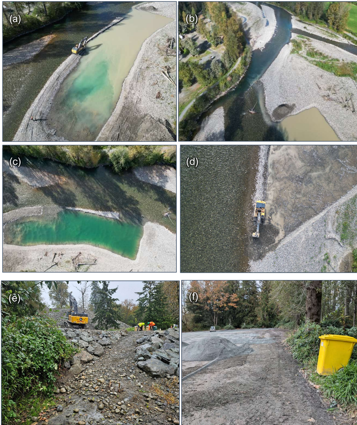
Figure 21. Photos taken at Lickman Bar by environmental monitors. (a) Excavation of upstream pit opening (Sep 20, 2024). (b) Outflow of turbid water from the downstream opening during the upstream opening (Sep 20, 2024). (c) Completed pit at Lickman Bar on Sep 23, 2024. (d) Opening of riffle enhancement area on Sep 23, 2024. (e) Restoration of the pedestrian ramp from the Rotary Trail to the bar top where the bridge had been installed (Sep 25, 2024). (f) Topping parking lot with crushed gravel after stockpiled material was removed (Oct 16, 2024).
