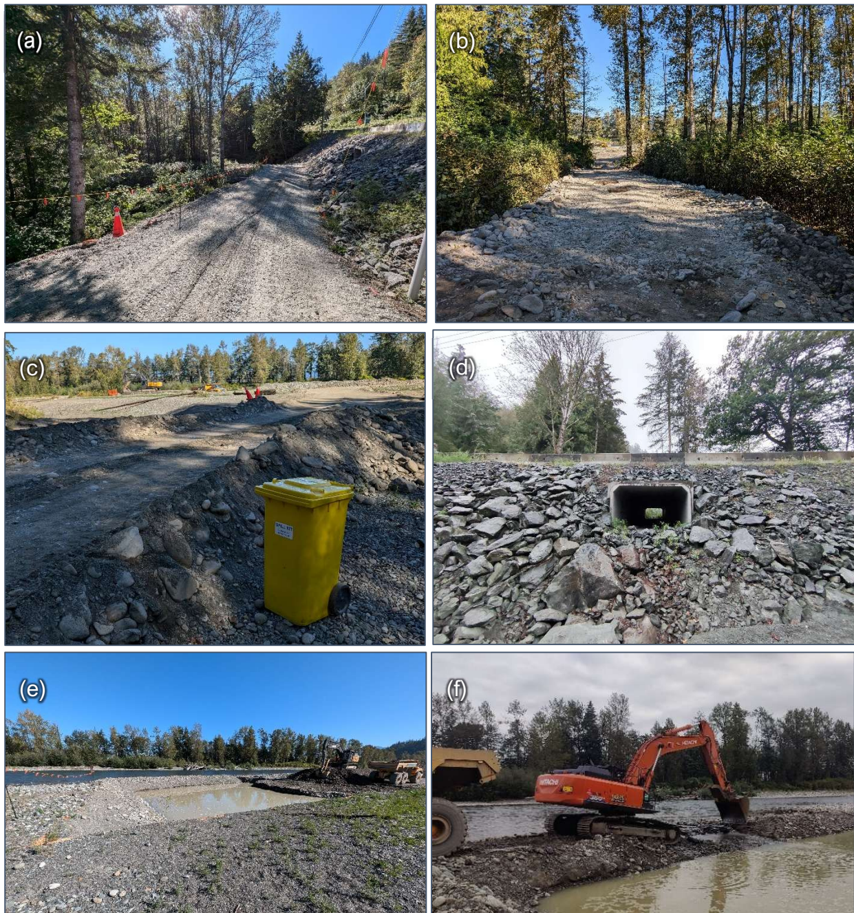
Figure 6. Photos of the works at S45 Bar by environmental monitors. (a) Access route along Rotary trail and culvert crossing (taken Aug 30 2024); (b) Access route where the access route departs from the Rotary Trail, looking toward the gravel bar (taken Aug 28, 2024); (c) Spill kit located on the gravel bar next to the access route (taken Aug 30 2024); (d) culvert under Vedder Mountain Road with no flow during rainy conditions (taken Sep 13). (e) Pit excavation at the downstream end (Aug 30, 2024). (f) Water flows into the pit during the downstream pit opening as water levels equalize (Sep 12, 2024).
