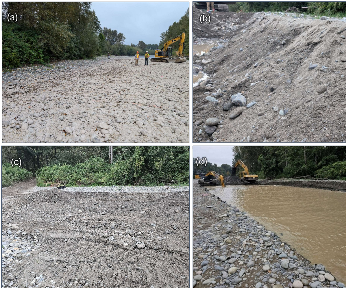
Figure 32. Photos taken at Bergman Bar by environmental monitors. (a) Preparing to dig a test trench for knotweed root search (Sep 2, 2024). (b) Inside wall of excavated trench (Sep 2, 2024). (c) Trench material was replaced and bar top material within the marked footprint was removed (Sep 2, 2024). (d) Bergman pit excavation (Sep 2, 2024).
