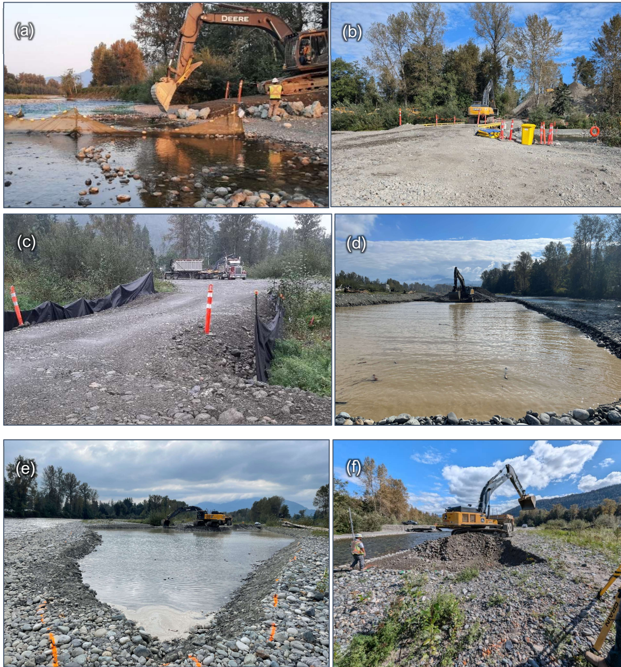
Figure 20. Photos of the works at Lickman Bar were taken by the environmental monitors. (a) Isolated and salvaged area for bridge abutment installation (Sep 6, 2024). (b) Completed bridge across from Lickman parking lot (Sep 9, 2024); (c) Geotextile and sediment was used to fill in a vegetated contour on the bar to allow access to the excavation site (Sep 13, 2024). (d) Downstream end of pit excavation (Sep 11, 2024). (e) Excavation of the upstream end of riffle excavation (Sep 18, 2024). (f) Downstream end of riffle excavation (Sep 17, 2024).
