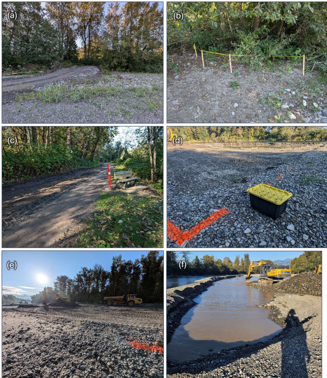
Figure 28. Photos taken at Brown Bar by environmental monitors. (a) Constructed access ramp (taken Aug 28, 2024). (b) Knotweed fenced off next to access ramp was undisturbed (Sep 5, 2024). (c) South Rotary Trail on Aug 28 2024. (d) Spill kit onsite next to excavation footprint (Aug 28, 2024). (e) Removal of top layer of gravel from pit footprint (taken Aug 28, 2024). (f) Pit excavation (Aug 29, 2024).
