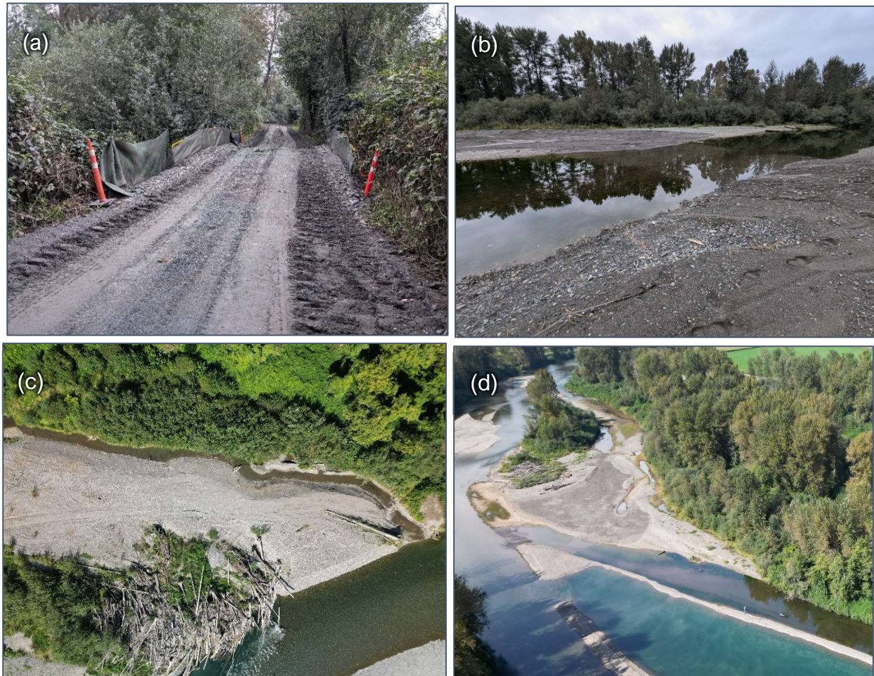
Figure 40. Photos of habitat enhancements at Greendale Bar. (a) Airbridge, geotextile and sediment placed overtop of a permanent bridge on the North Rotary Trail for bar access (Sep 12, 2024); (b) Airbridge removed from side channel crossing location (Sep 18, 2024). (c) Completed microchannel excavation and LWD installations at upstream end of Greendale Bar (Sep 18, 2024). (d) Completed bar top removal at downstream end of Greendale Bar (Sep 18, 2024).
