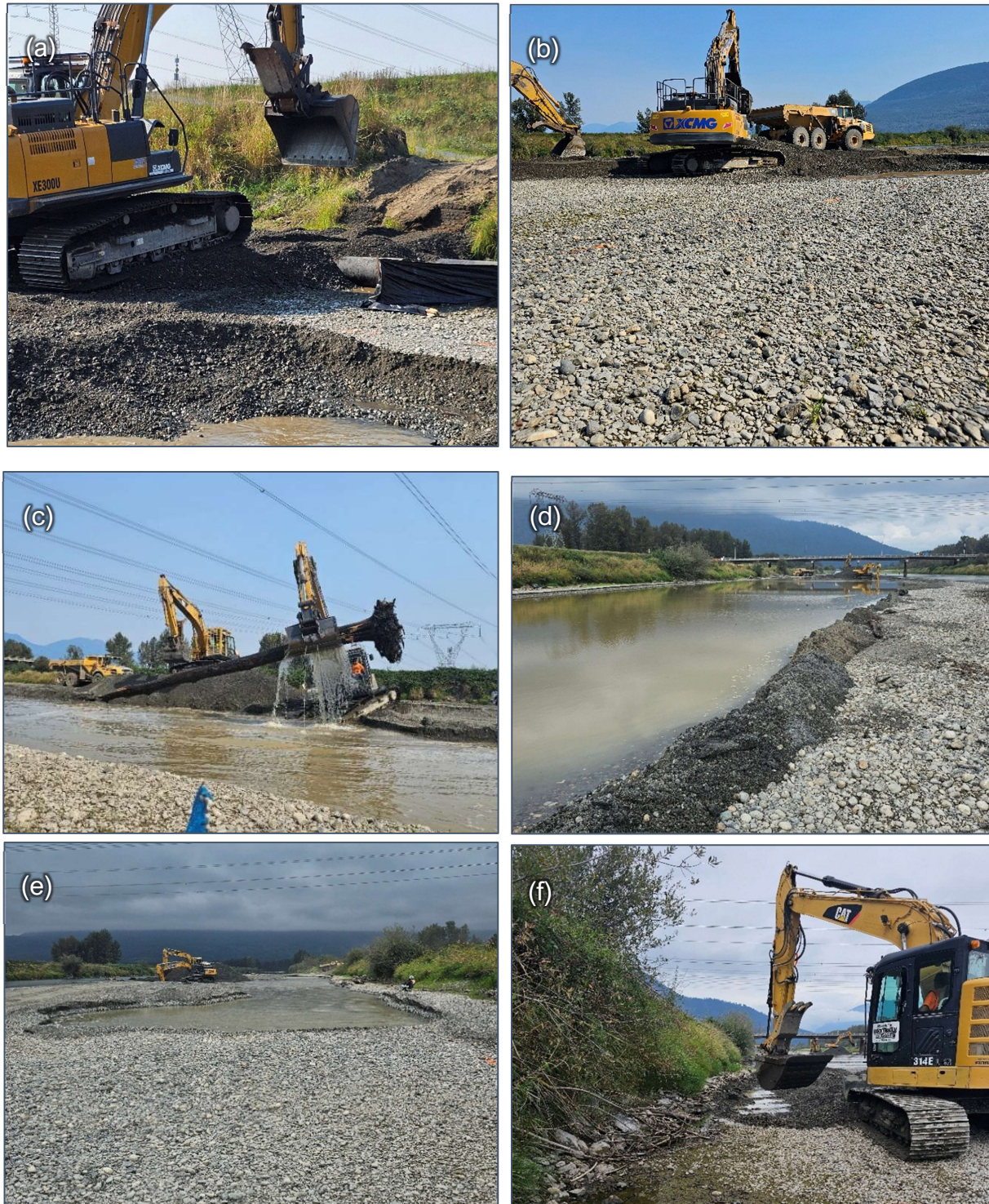
Figure 45. Photos taken by environmental monitors at Powerline Bar. (a) Silt curtain downstream of the access ramp and within the salvages area (Sep 6, 2024). (b) Pit excavation began on Sep 6, 2024. (c) Piece of LWD recovered during pit excavation (Sep 7, 2024). (d) Berm around pit (Sep 13, 2024). (e) Pit excavation at upstream end of the bar (taken Sep 10, 2024). (f) Sediment added to the berm between the pit and side channel along the left bank (taken Sep 10).
