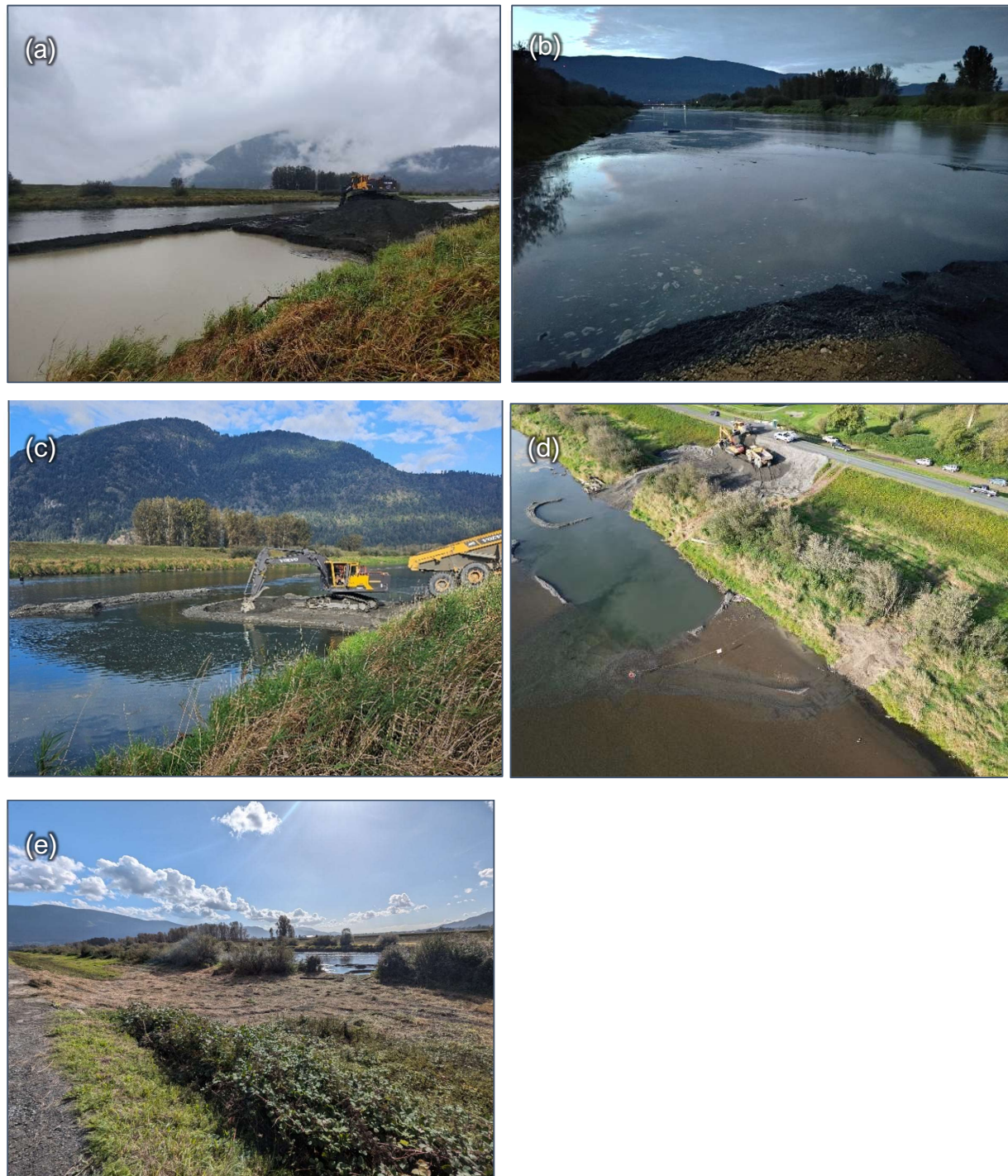
Figure 50. Photos taken at Chadsey Bar by environmental monitors. (a) Berm has been added around the full perimeter of the pit and stockpiled material at the access ramp was being removed on Sep 25, 2024. (b) Berm overtopped on the morning of Sep 26, 2024. (c) Excavation of the middle cell of the pit on Sep 26, 2024. (d) Aerial photo of the upstream end of Chadsey Bar after all openings were complete (Sept 27, 2024). (e) Dike slope and bench after geotextile was removed and site was fully decommissioned (Oct 4, 2024).
