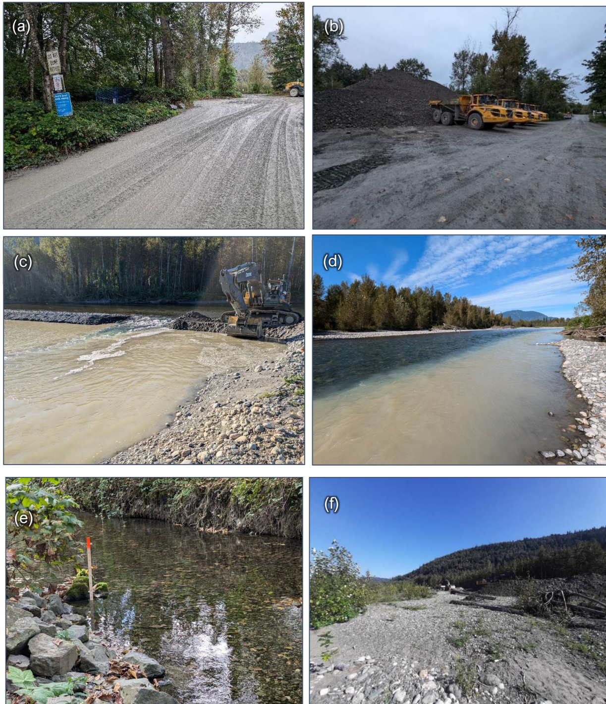
Figure 16. Photos taken by environmental monitors at Peach Road Bar. (a) No runoff issues along the hauling route near the Peach Creek Spawning Channels during rain on Sep 11, 2024. (b) Stockpile and machinery at the Lickman parking lot (taken Sep 10, 2024). (c) Downstream pit opening on Sep 16, 2024. (d) Turbid water travelling along bar edge 20 m downstream during pit opening (Sep 16, 2024). (e) No impacts to water levels detected at temporary staff gauge installed in Peach Creek Spawning Channel on Sep 17, 2024. (f) Restored bar top (Sep 19, 2024).
