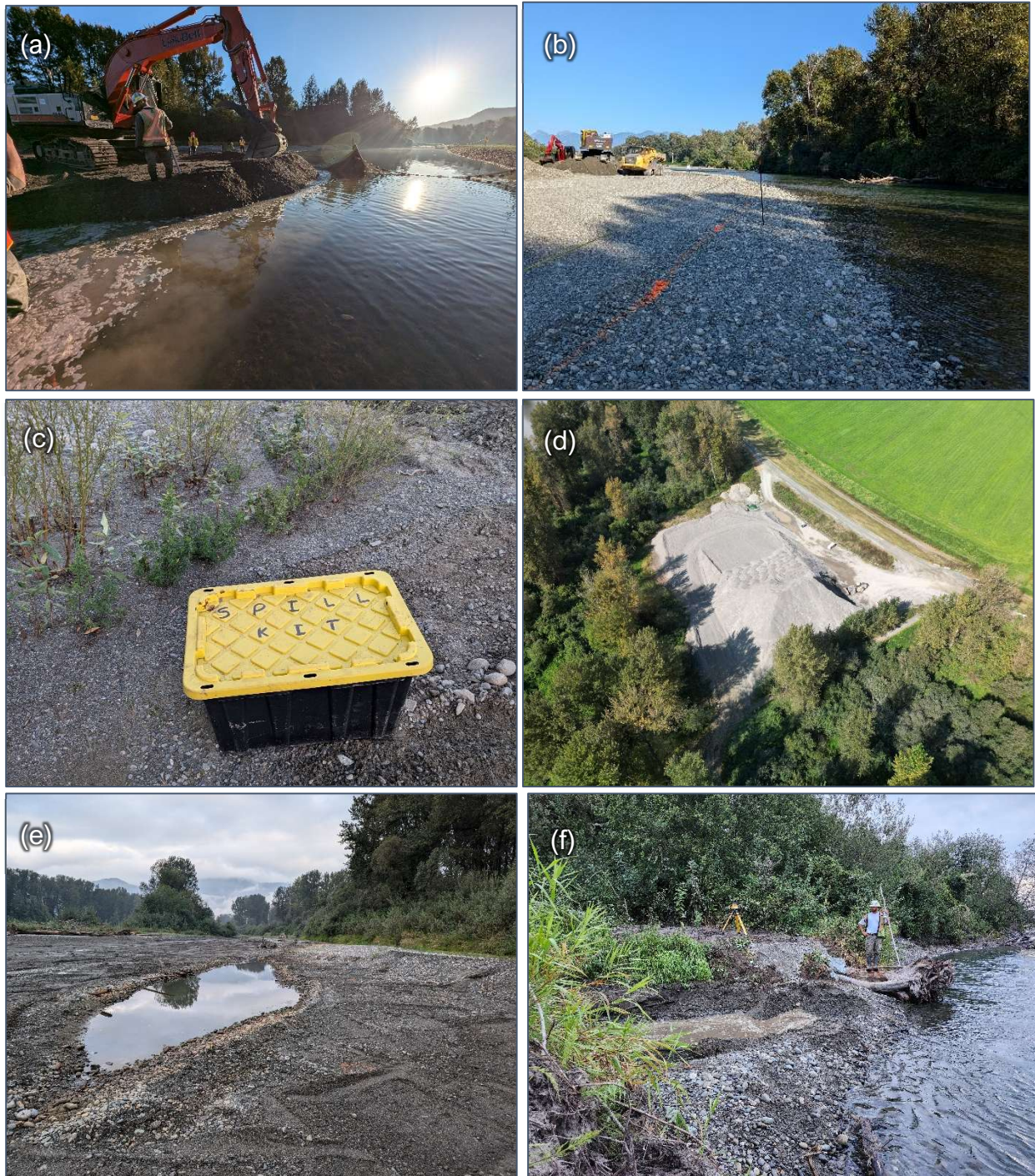
Figure 39. Photos taken at Greendale Bar by environmental monitors. (a) Completed base of sediment for side channel crossing within isolated area lined with silt curtain at upstream and downstream ends (taken Aug 28, 2024); (b) Main channel during pit excavation (taken Aug 30, 2024). (c) Spill kit onsite during excavations (taken Aug 31, 2024). (d) Bar top removal did not disturb the remnant pool in the center of the bar (taken Sep 12, 2024). (e) Side channel crossing location after airbridge was removed (taken Sep 12, 2024).
