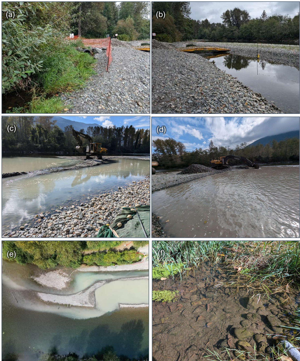
Figure 36. Photos taken at Railway Bar by environmental monitors. (a) Snow fencing placed around culvert and knotweed and spill kit (Sep 11, 2024). (b) Airbridge installed over backwater for site access (Sep 11, 2024). (c) The berm started to breach as the excavator accessed the bar to complete the downstream opening (Sep 17, 2024). (d) Completed upstream opening at 12:20 pm on Sep 17, 2024; (e) Aerial photo of pit following completion of both openings on Sep 17, 2024. (f) No turbidity reached culvert outflow (Sep 17, 2024).
