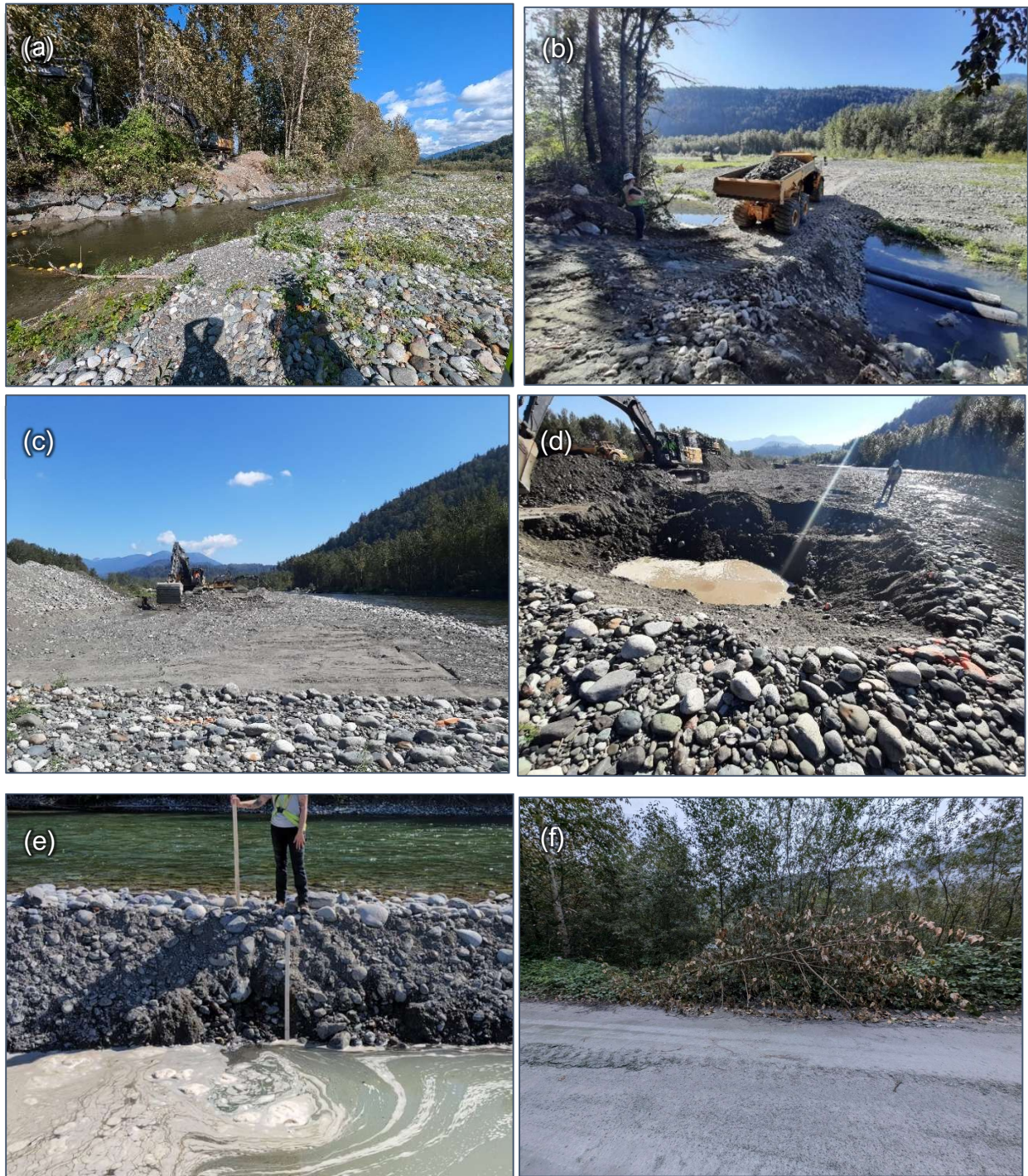
Figure 15. Photos taken by environmental monitors at Peach Road Bar. (a) Culverts placed at the toe of the bank within an isolated and salvaged area prior to ramp construction (Aug 27, 2024). (b) Access ramp nearly complete (Aug 27, 2024). (c) Stockpiling of bar top material prior to deep excavation at Peach Bar (Aug 28, 2024). (d) Pit is slow to fill with water once deep excavation begins (Aug 29, 2024). (e) Spring of water from main channel causing some erosion (Aug 30, 2024). (f) Tree found next to Rotary Trail along the access route appeared to have been felled by a beaver (Sep 11, 2024).
