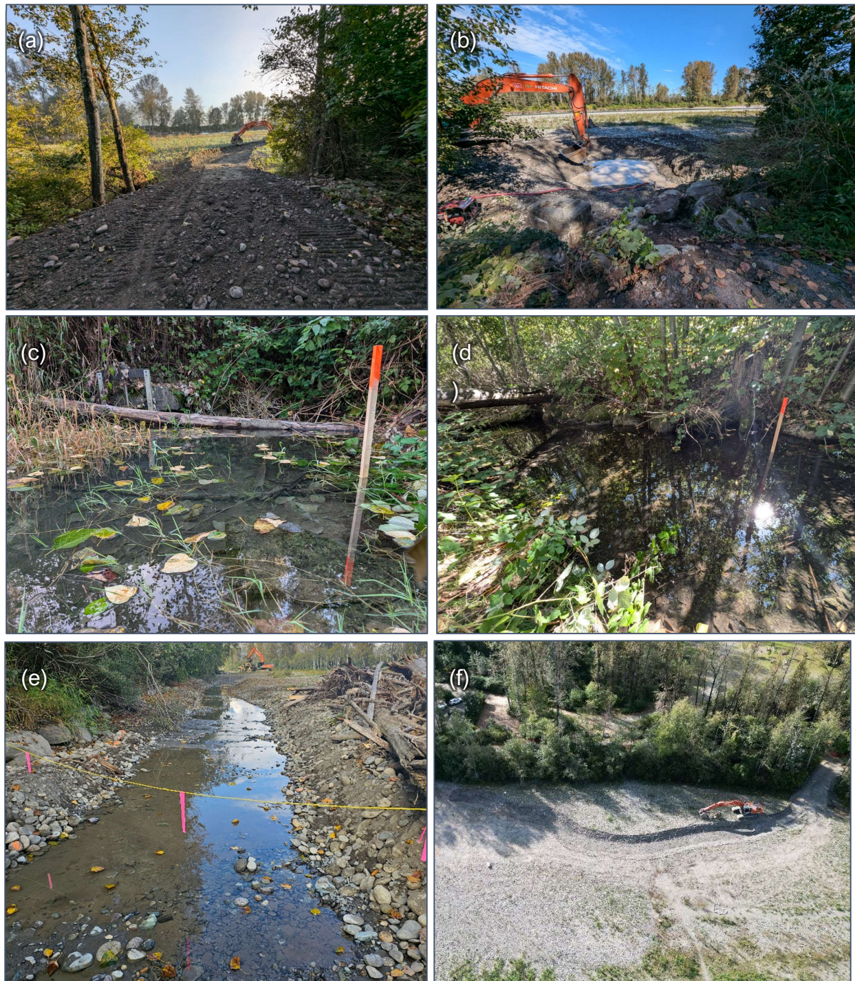
Figure 23. Photos taken at Campground Bar by environmental monitors. (a) Access ramp onto the bar (taken Sep 17, 2024). (b) Small pit was excavated at the pipe intake on Sep 16, 2024, and a small water pump controlled the water level. (c) Staff gauge marking the upstream monitoring location for wetland enhancement (Sep 17, 2024). (d) Staff gauge marking the second monitoring location 120 m downstream (Sep 17, 2024). (e) Excavation at upstream end where water is seeping in prior to removing the berm at the upstream end (Sep 19, 2024). (f) Aerial drone image of habitat enhancement channel and access ramp (Sep 21, 2024).
