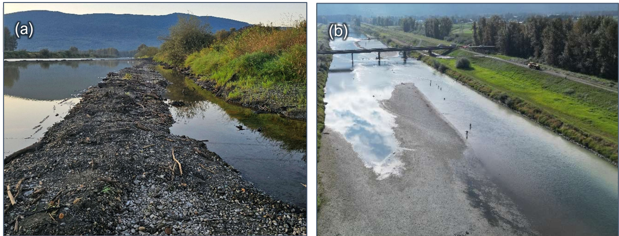
Figure 46. Photos of the works at Powerline Bar by environmental monitors. (a) Completed microchannel at upstream end (Sep 16, 2024). (b) Turbid water from Powerline Bar pit opening moving along the left bank on Sep 17, 2024.
