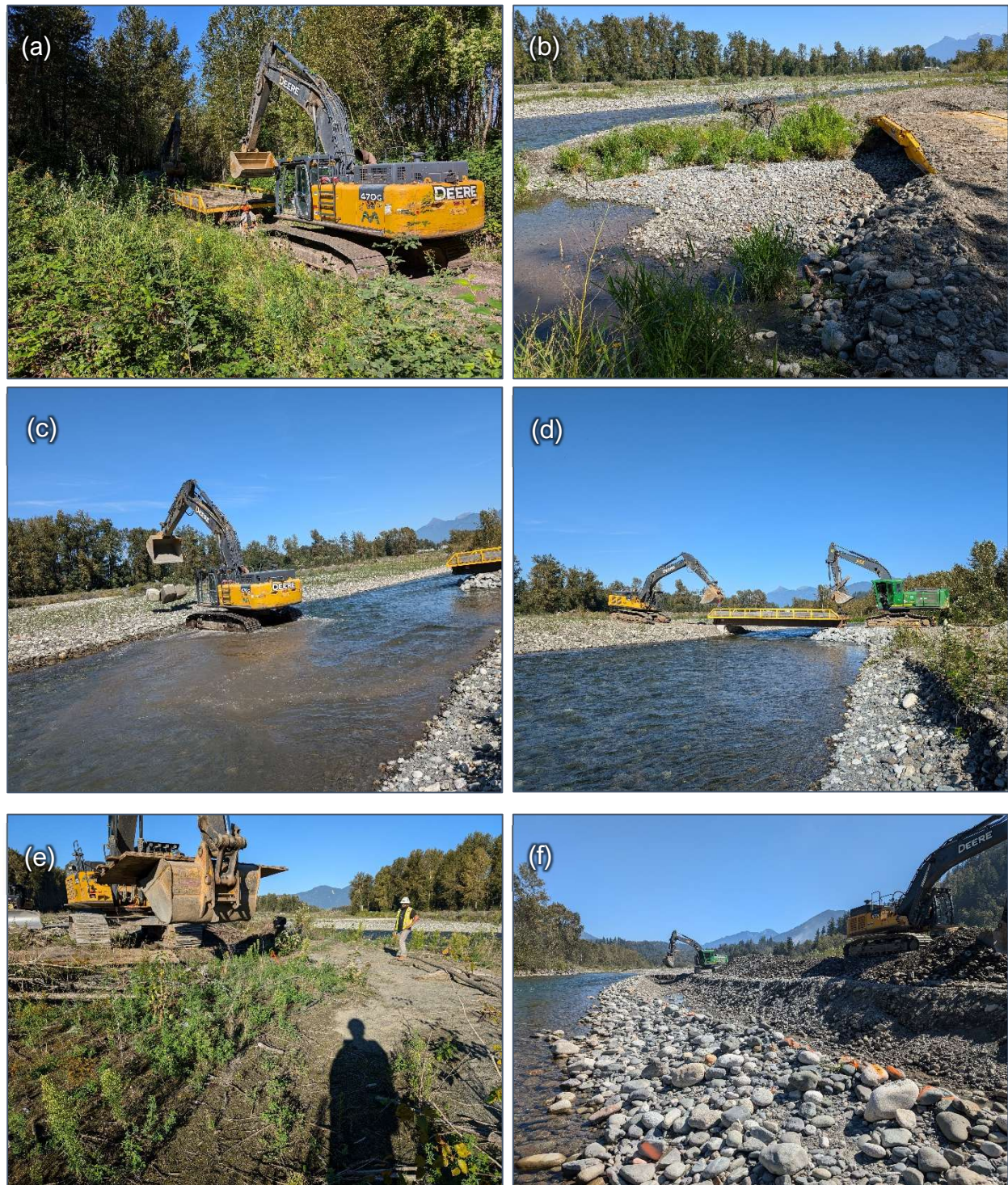
Figure 10. Photos taken at Giesbrecht Bar by environmental monitors. (a) Excavators carrying bridge to the river bank via the existing trail (taken Aug 27, 2024). (b) Side channel running dry after the installation of airbridge (taken Aug 28 2024). (c) An excavator completed one wet crossing to construct the side channel crossing (taken Aug 29 2024); (d) Bridge was moved into place by excavators positioned on land (taken Aug 29 2024). (e) Access route established along the bar top (taken Aug 30 2024); (f) Pit excavation was completed in lengthwise stripes and briefly stockpiled in windrows behind the excavator within the pit footprint (taken Aug 30 2024).
