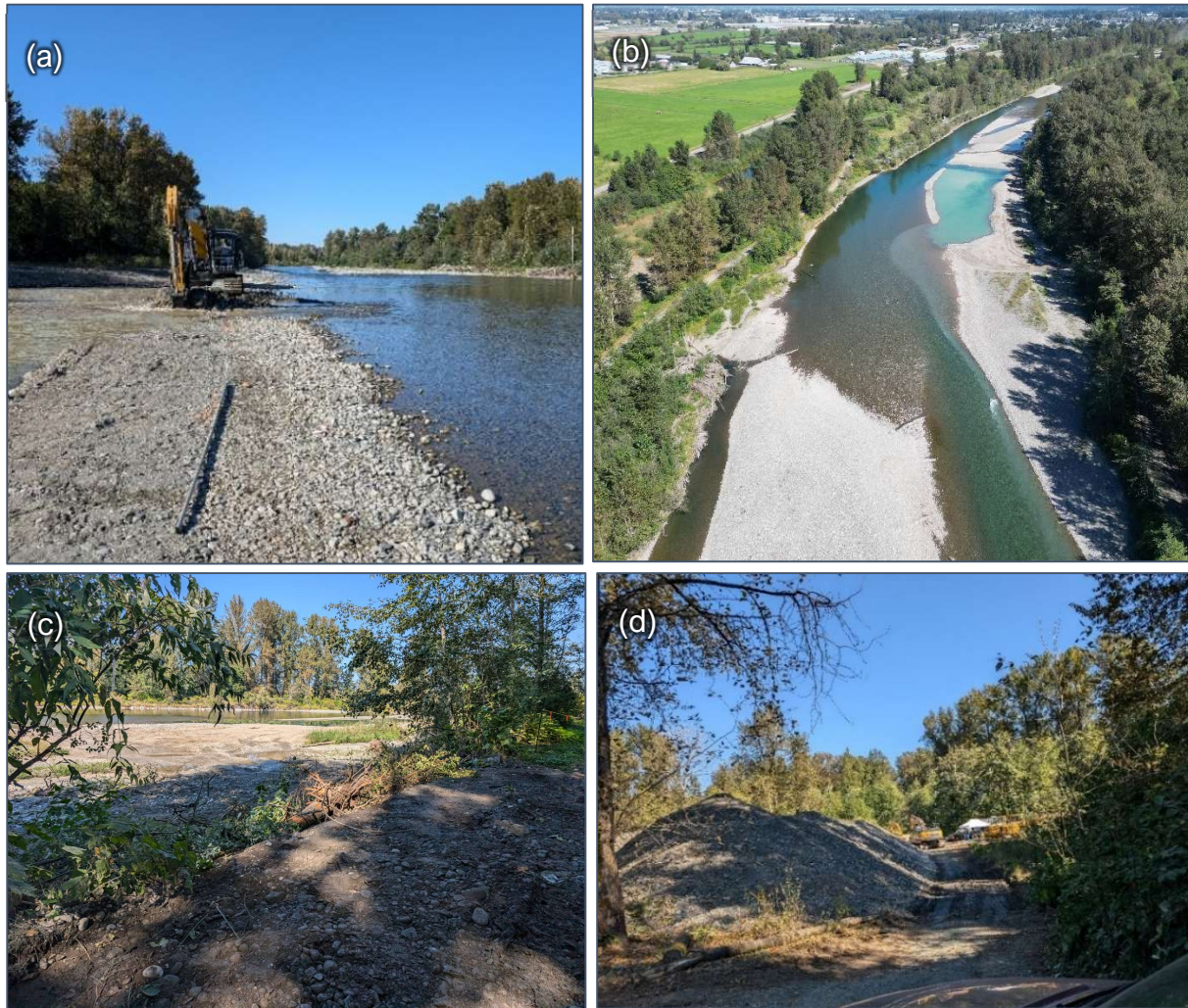
Figure 29. Photos taken at Brown Bar by environmental monitors. (a) Downstream pit opening at Brown Bar on Sep 5, 2024. (b) Aerial photo of pit and bar top removal after openings were completed (taken Sep 5 2024). (c) Access ramp area restored (Sep 6, 2024). (d) Bergman stockpile (Oct 4, 2024).
