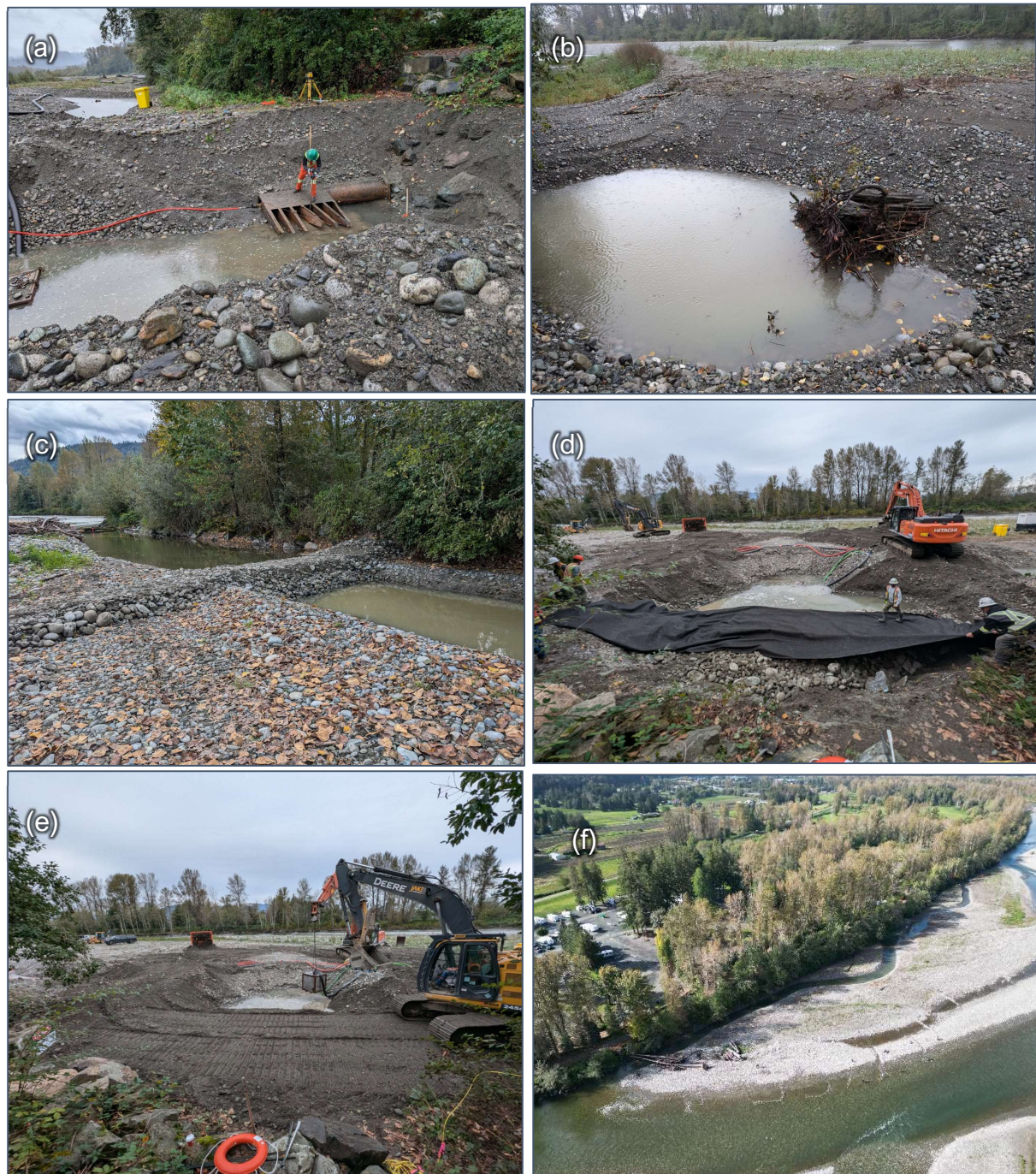
Figure 24. Photos taken at Campground Bar by environmental monitors. (a) Two berms at the upstream end of the enhancement excavation (Sep 26 2024); (b) LWD placement within one of the pools in the habitat enhancement excavation (Sep 24, 2024). (c) CCTV inspection of the pipe on Sep 25 2024; (d) geotextile laid over large cobble during construction of the infiltration gallery (Sep 26, 2024); (e) excavator packing the finer sediment over the infiltration gallery. (f) Aerial photo of completed habitat enhancement excavation connected to the main channel at the upstream and downstream end of Campground Bar (Sep 28, 2024).
